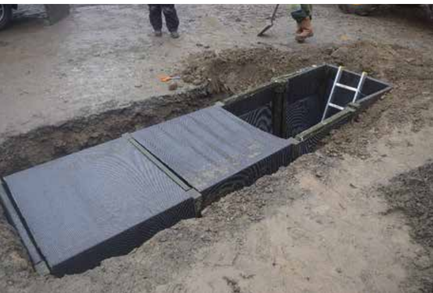
▲ The Universal Battle Trench shown here is designed to be carried on a standard pallet and added to pre-positioned equipment so that it can be quickly deployed in the event of war. It provides greater protection and structural strength than a standard trench. [B+SL]
